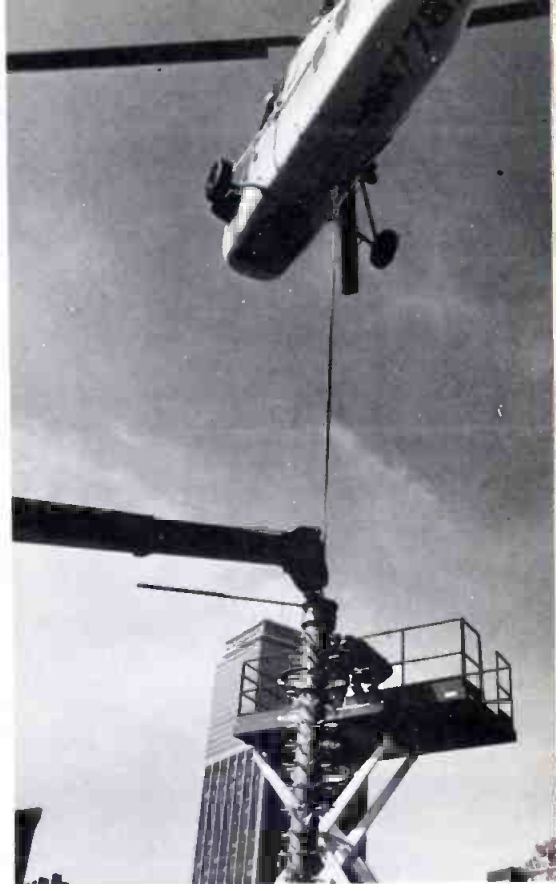
Spiral antenna bay is tilted vertical and technician attaches cable to hovering helicopter.
